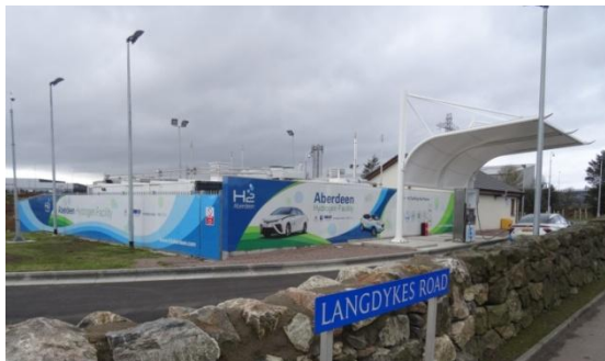
ACHES 350/700 bar hydrogen refueling station, Aberdeen (UK)
