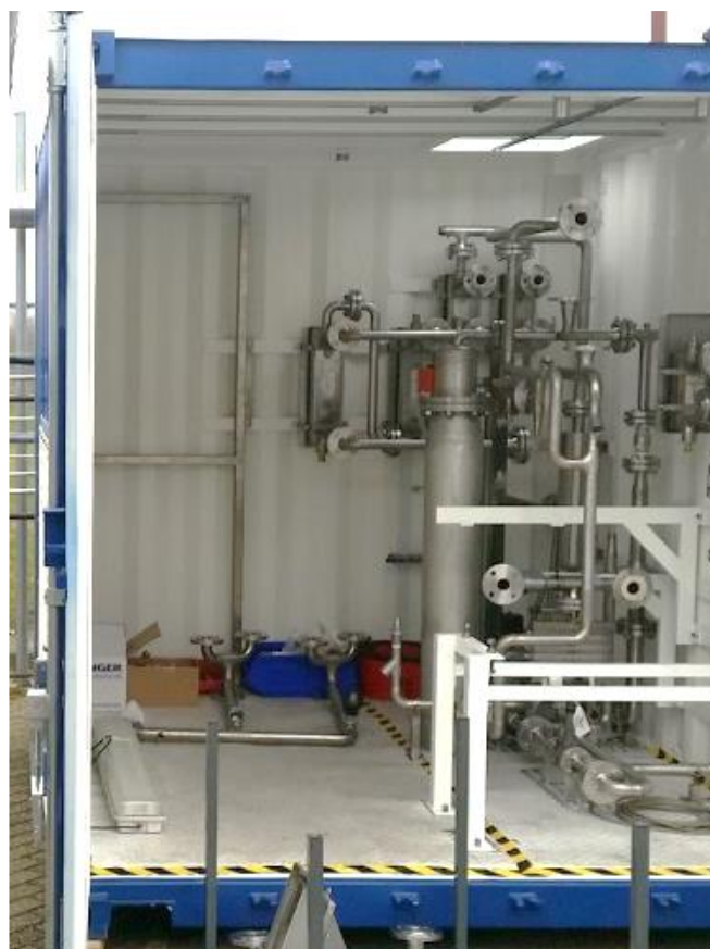
Figure 9. TSA pilot plant under construction.
